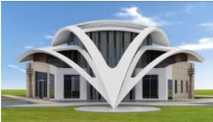
(A Banglow in Noida, elevation in ferrocement)
