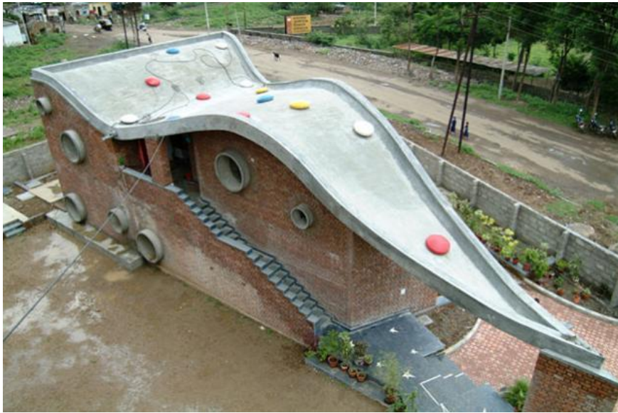
(Lahuji Vastad Health Centre Aurangabad with ferrocement roof)
