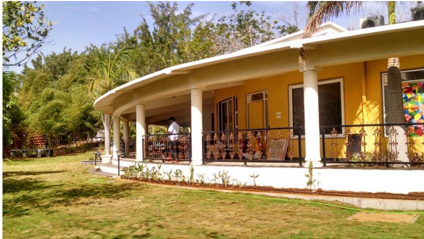
(A Banglow near Bhugaon, built by Padmanabh Lele)
