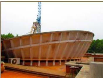
Largest Solar Kitchen in South Asia at Auroville, India Solar collector is made with ferrocement.
