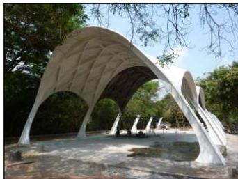
Ferrocement component casting yard at CSR Auroville, near Puducherry. Width is 14 metre and the height is 7 meter. Many ferrocement structures implemented by Auroville Centre for Scientific Research (CSR) are testimony of durability of the ferrocement technology
