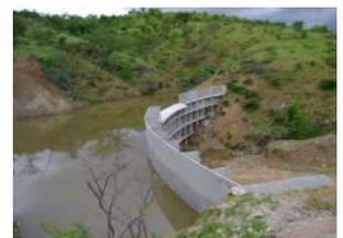
Margarito Ortiz Gumán from Oaxaca, Mexico has built a 6m high and 27 m wide ferrocement dam in 2010. The thickness is 50 mm. The dam is useful for drinking water, irrigation and to recharge the water table in arid area.
