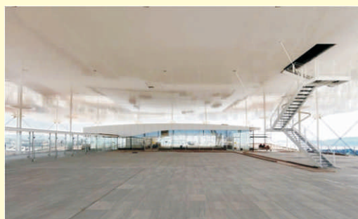
The largest ferro-cement span in the world ... underneath the cultural centre's canopy. Photograph: Michel Denancé
