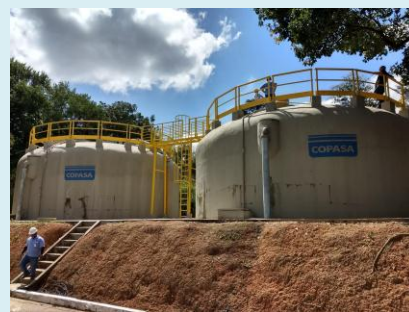
Figura 2 - The two recovered UASB reactors
